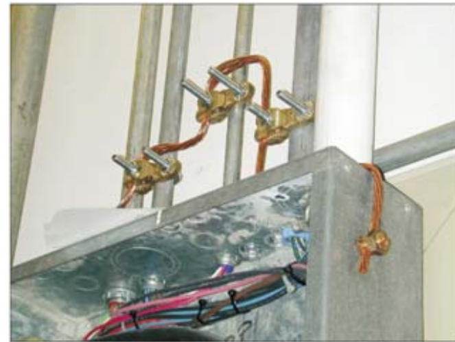
FIGURE 1-7 Bonding conduits to panelboard cabinet
