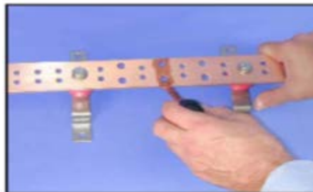
Applying an antioxidant to the cleaned area of the grounding busbar
