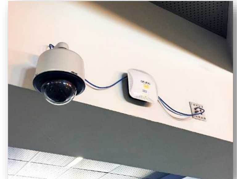
Photo taken at McCarran Airport in Las Vegas – Anyone could jump up and pull out the patch cord to the surveillance camera and wireless access point.
