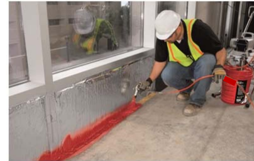
Edge of Slab Joints
