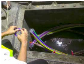
Smaller Ducts & Handholes
